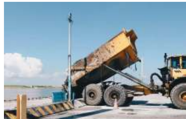
The ash being treated at Semakau before discharged as water into the open sea.
